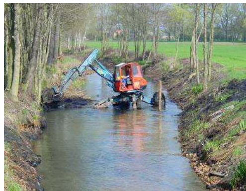
Abb. 3 Entschlammung [39]
